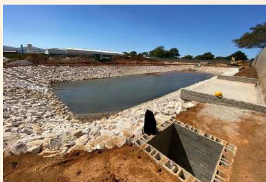
Overflow channel for water treatment pond at Coca-Cola plant Lusaka west
