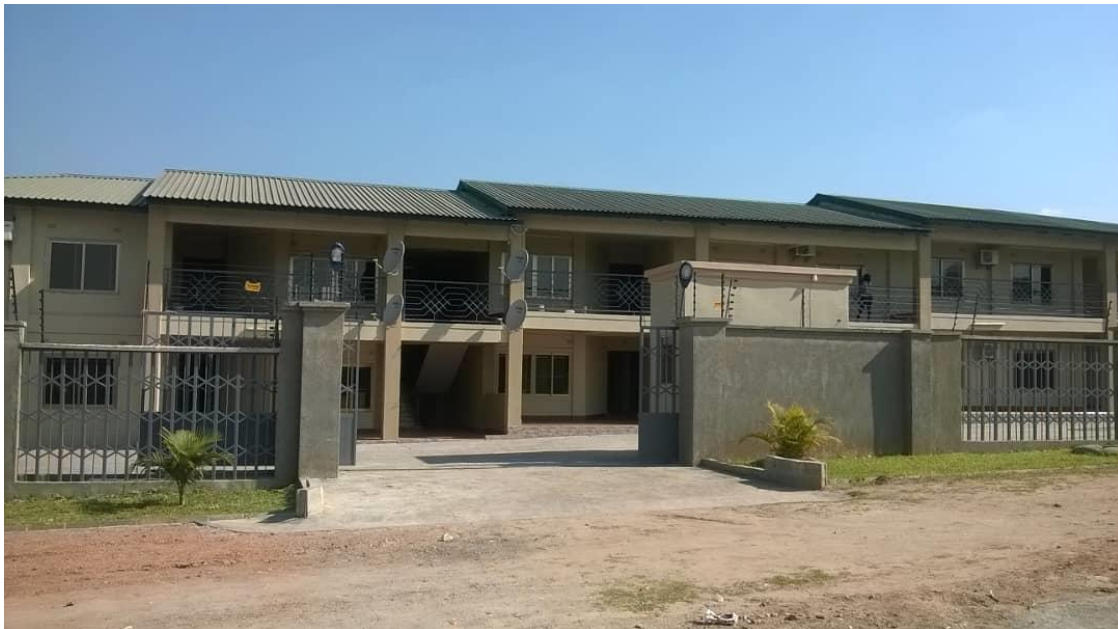
Figure 9 Block of Flats constructed for an individual client in Kitwe Copperbelt Zambia
