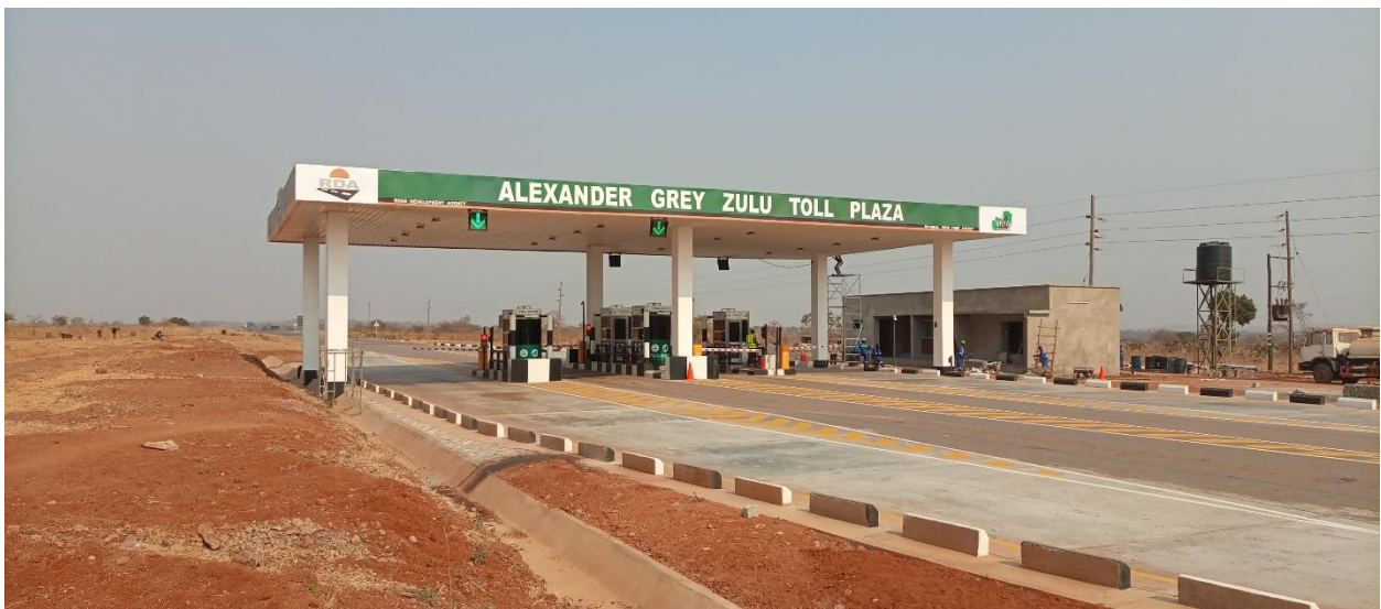
Figure 6 Toll Gate infrastructure carried out by PCA Civils for the Road Development Agency - RDA
