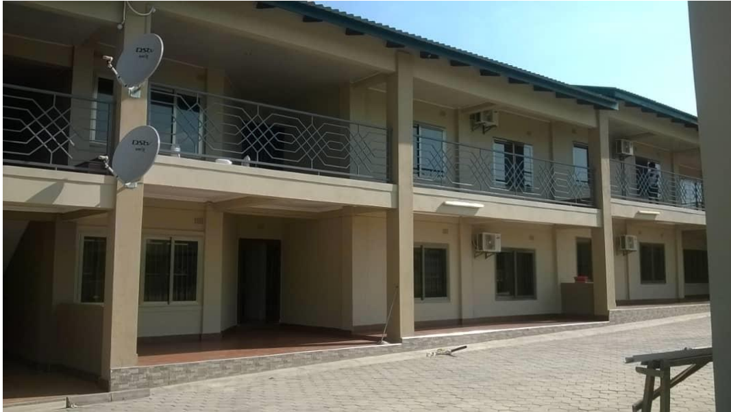
Figure 8 Block of Flats Constructed for an individual client in Kitwe
