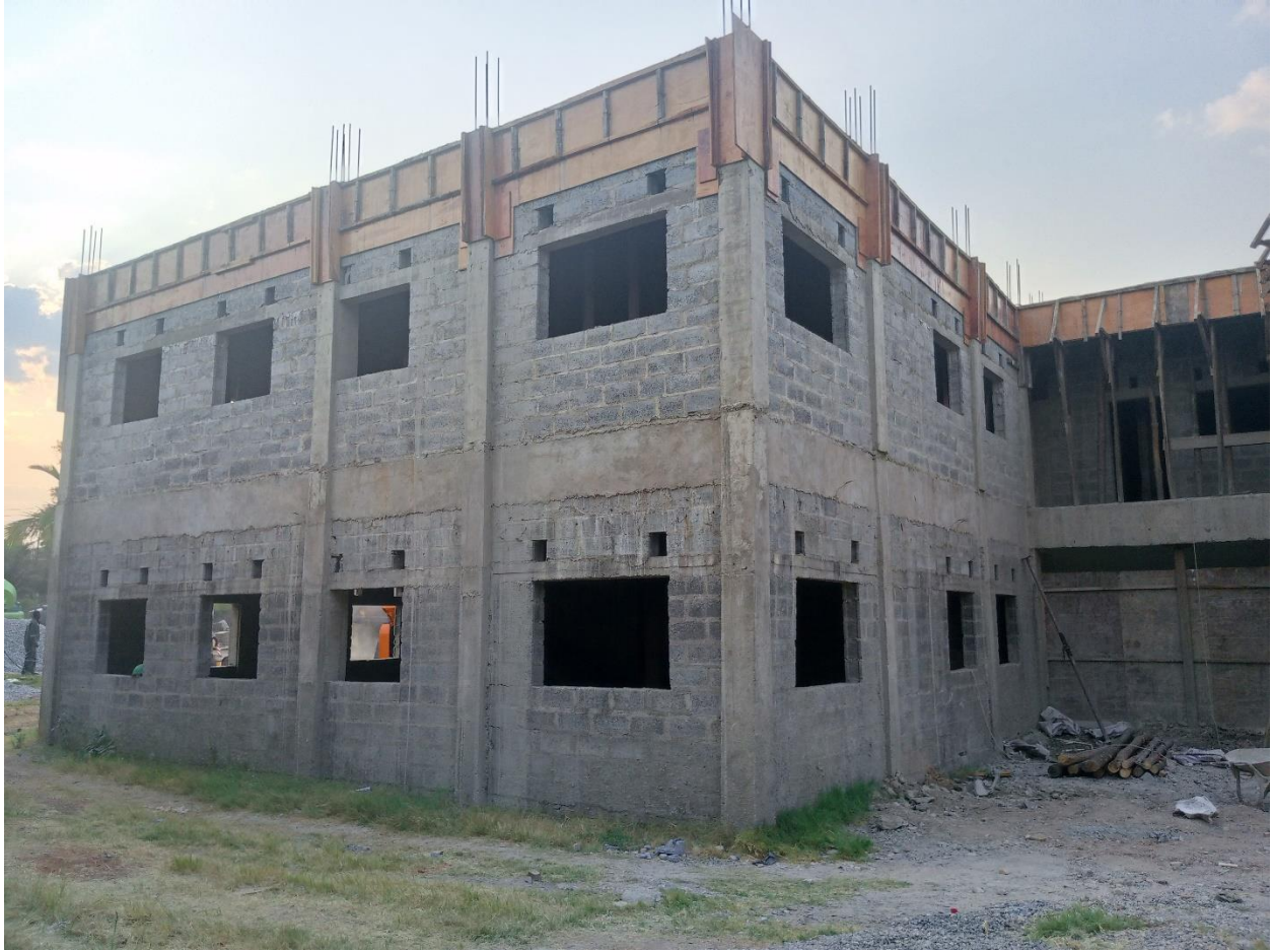
Figure 10 Construction of School Infrastructure by PCA Civils Ltd in Kitwe
