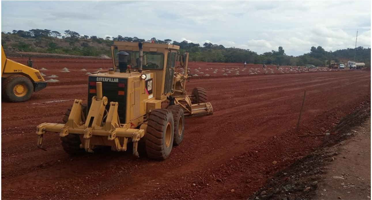
Figure 5 Earthworks carried out by PCA Civils
