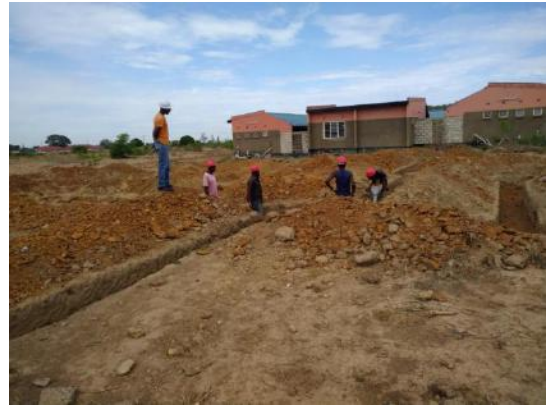
Setting-out & Foundation Trench Excavation
