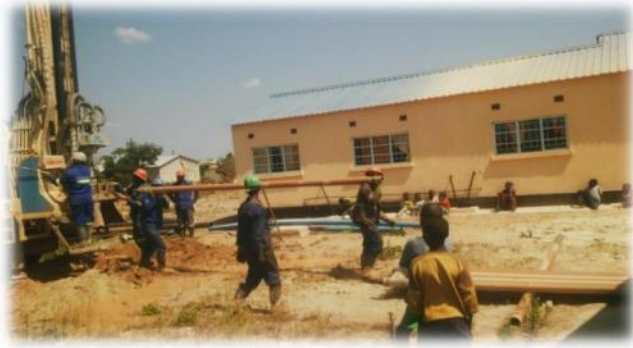
Right- Drilling of Borehole at Musumali RHC.
