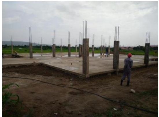
Sub-structure Slab and Super-structural Pillars
