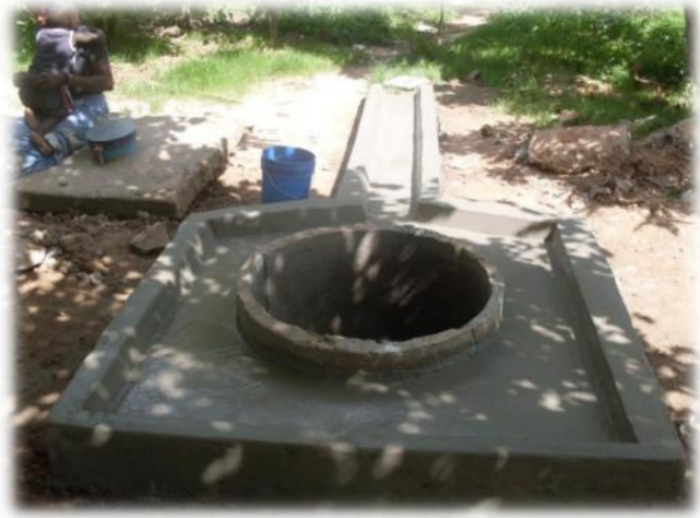
Right: Shallow well under Construction
