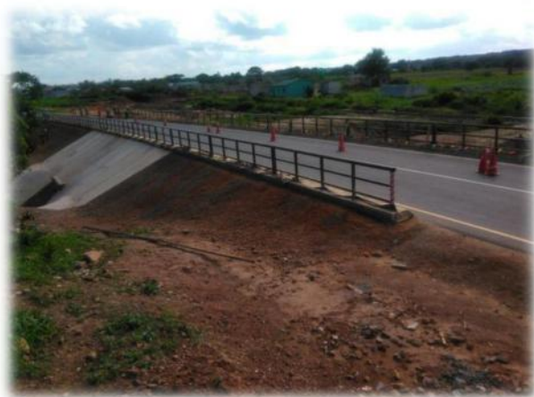
Protection & Guardrail installation just completed
