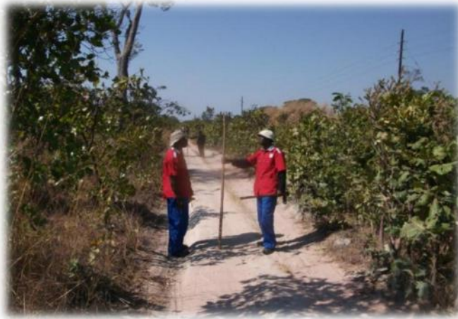
Left: setting-out and Road alignment.
