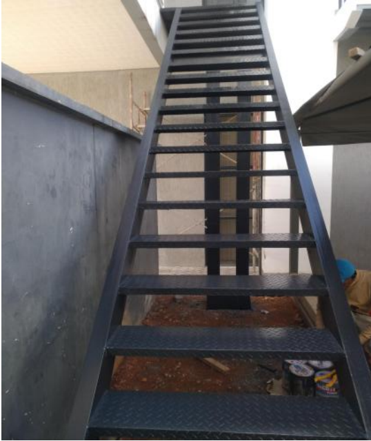
Fabrication of Steel Fire Escape Staircase
