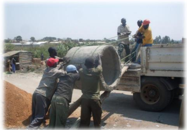
CAIP PROJECT: 900mm and 600mm Ring culverts ready for to the Mansa Municipal Council for CAIP Projects. July, 2011
