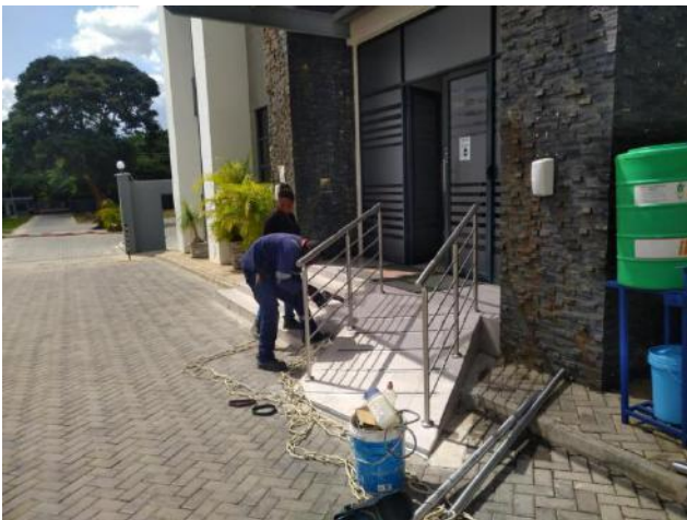
Stainless Steel Guard-rails installation & finalising the reconstruction of the Frontage of Buildings
