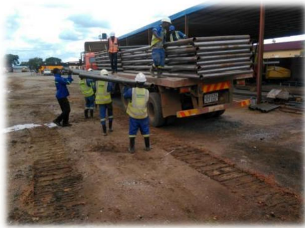
Loading Of Guardrails from the Fabricating bay
