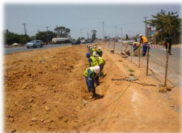
Drainage Excavation
