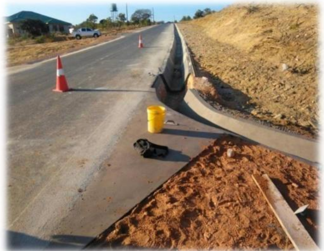
Newly Casted Concrete Drain
