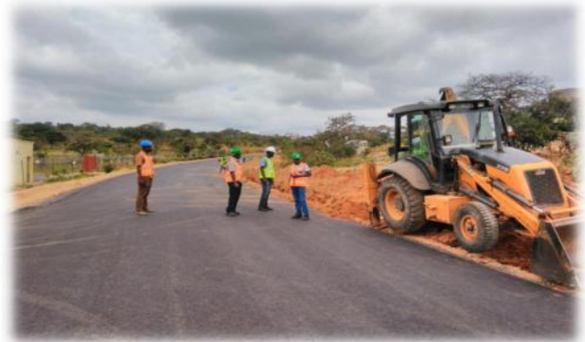
Excavation of a --- Drainage
