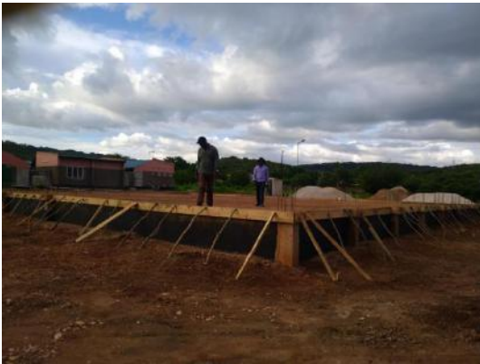
Compacted Foundation Box
