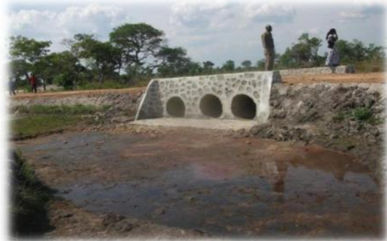
Embarkment and Culverts Installed at Chibinda swampy area, part of the source of Mansa River.
