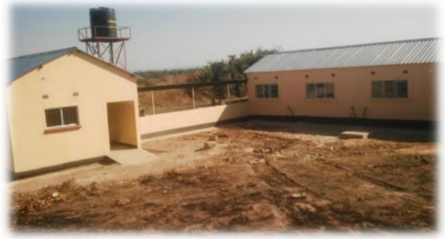
Right- The just completed Sumbu RHC
