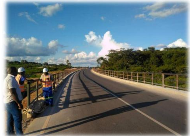
Protection & Guardrail installation just completed
