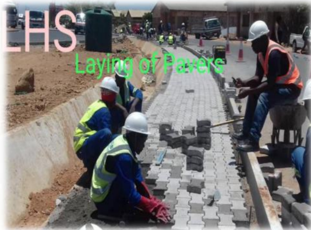
900mmX 600mm Trapezoidal Drainage & Walkway Paving at S.OS Roundabout of the Great East Road Completed- October 2019
