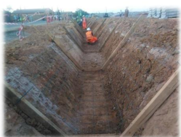
Drainage shaped & Templates set out in
