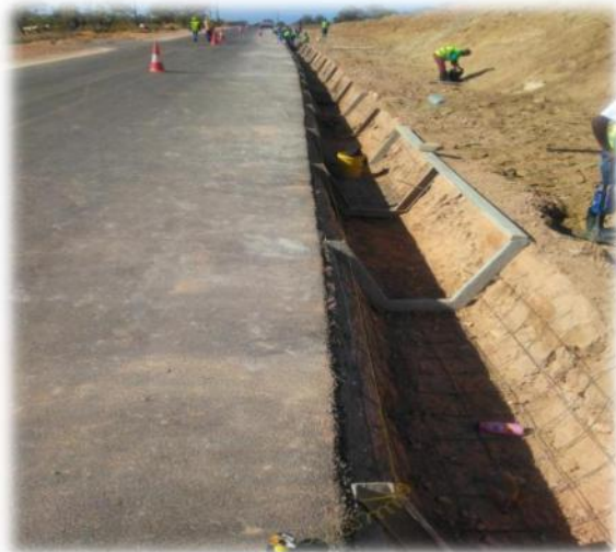
Drainage shaped & Templates set out in readiness to receive concrete
