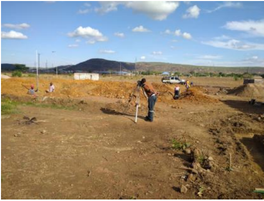
Setting-out & Foundation Trench Excavation
