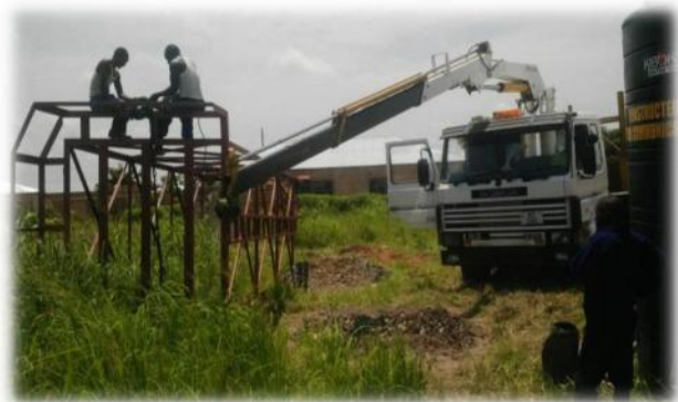
Erection of water Tank Stand at Musomali RHC
