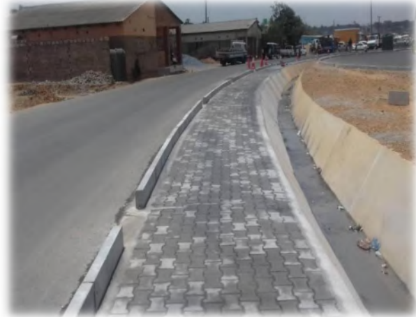
900mmX 600mm Trapezoidal Drainage & Walkway Paving at S.OS Roundabout of the Great East Road Completed- October 2019
