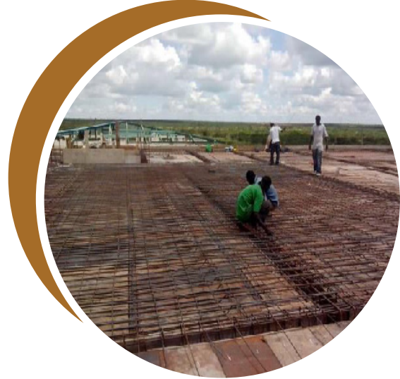
Steel Fixing
