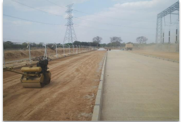
CONCRETE ROAD AND LAND PREPARATION
