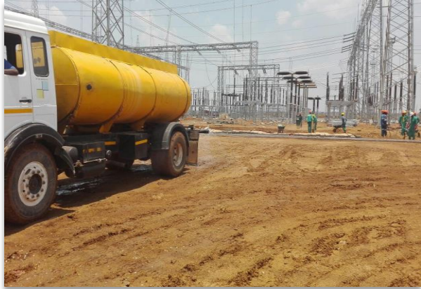
GROUND PREPARATION WORKS ZESCO SUB STATION LUSAKA WEST
