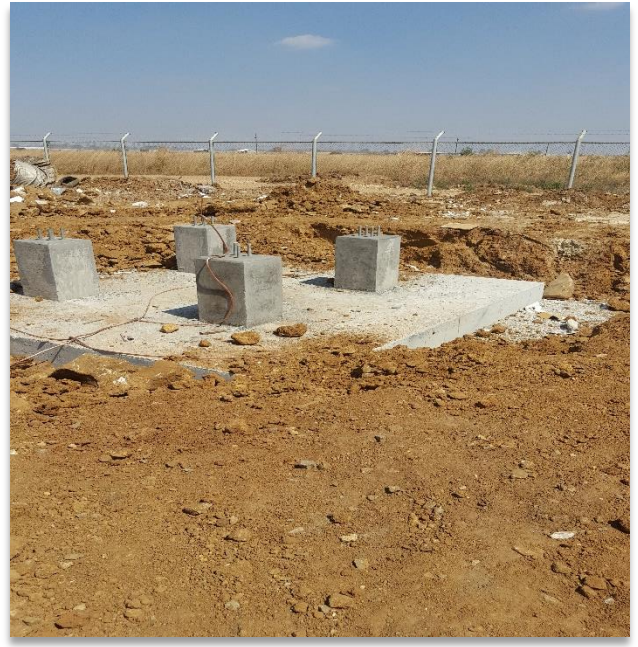
SUPPORT FOR SUBSTATION EQUIPMENT ( PLINTH)
