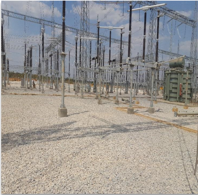
SUPPLY AND SPREADING OF 20MM TO 40MM STONE ZESCO SUBSTATION MUMBWA 18000 TONS
