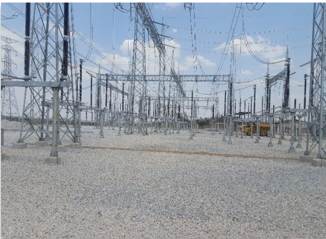
SUPPLY AND SPREADING OF 20MM TO 40MM STONE ZESCO SUBSTATION MUMBWA 18000 TONS
