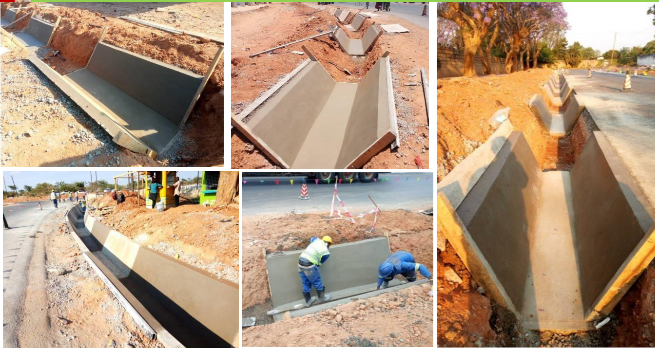
Construction of Trapezoidal Concrete Drainages (AVIC International – Lusaka, 2018)
