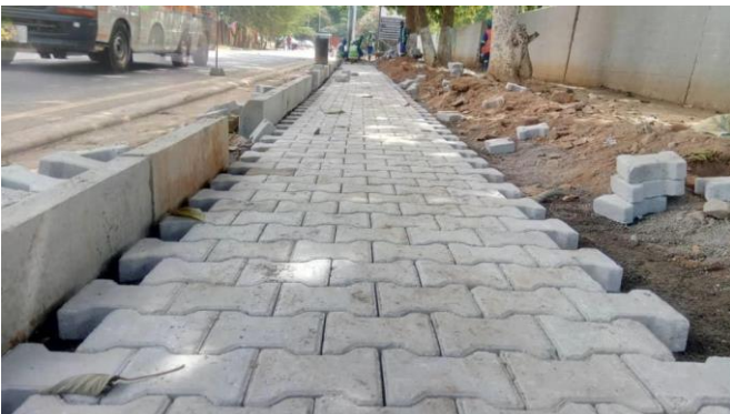
Side walk and Kerb Stones constructions ((AVIC International – Lusaka, 2018)
