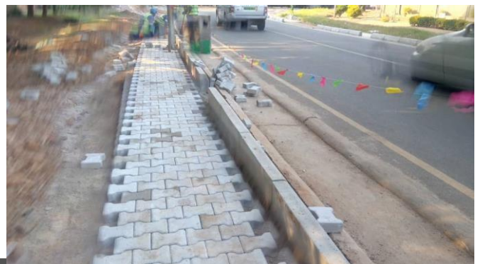
Side walk and Kerb Stones constructions ((AVIC International – Lusaka, 2018)
