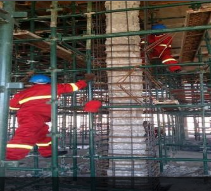
Skilled Scaffolders erecting scaffolds (Cosmopolitan Mall Project, 2015)
