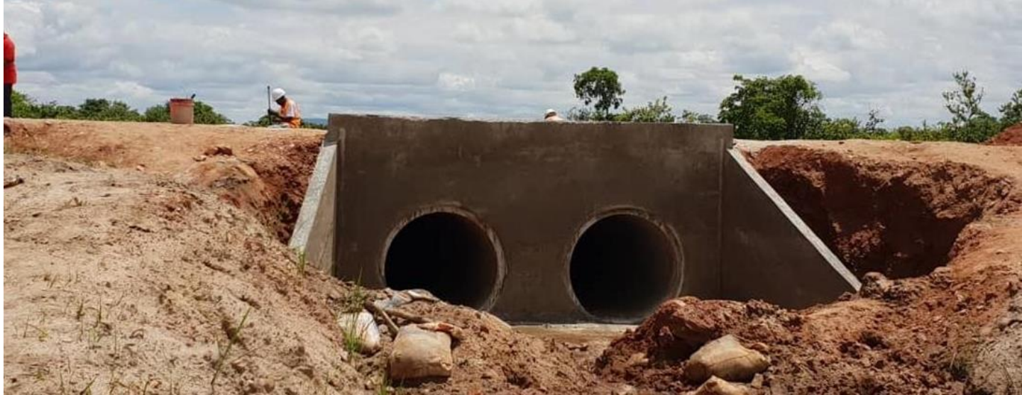
Drainage construction using stone pitching (RDA/Gomes – Ndola , 2014)
