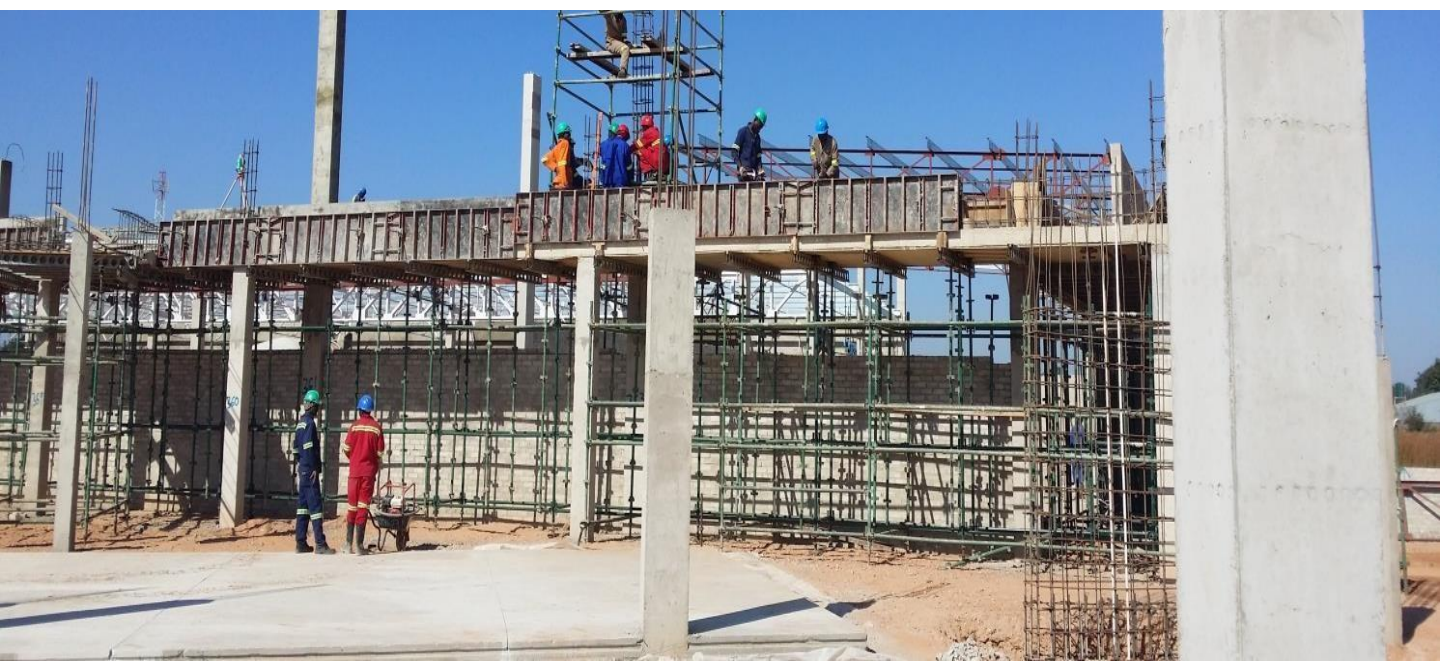
Construction of Cosmopolitan Mall (Lusaka, 2015)
