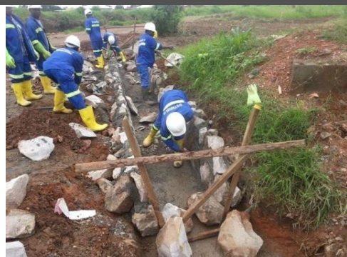
General workers helping the bricklayers (RDA Project, 2013)
