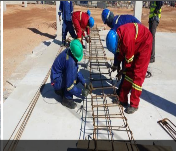
Steel fixers on hired labour (ZBL Project, 2015)
