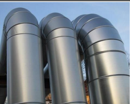
Products of our highly skilled sheet metal developers (Thermal Insulation)
