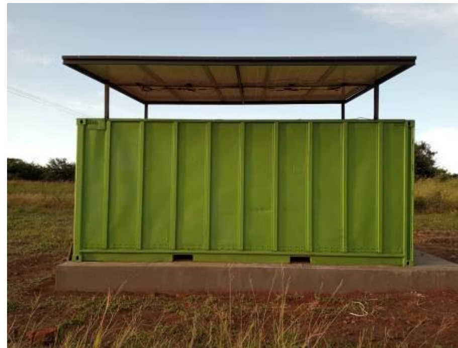
Solar Cold-Room In Mpunde - Kabwe Rural
