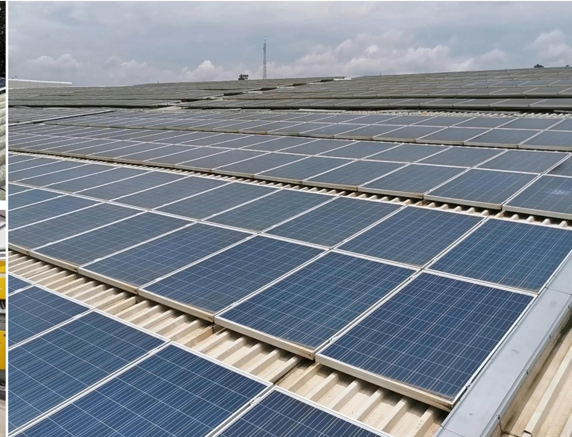
240KW Grid Connected Solar System for Medical Stores
